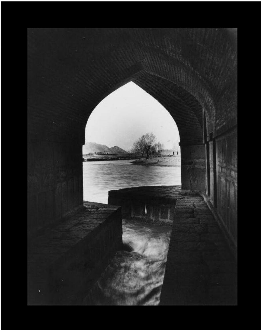
Figure 19. The sluice gate under the bridge. The sluice gate is located under octagonal pavilion called "Byglrbygy" (photograph by Robert Byron [1905-1941], 1933-1934).
